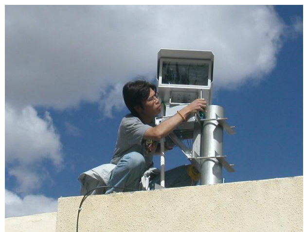
Flexible deployment options include Pole-mount installation of CableFree FSO units. Wide-beam optics makes tower deployments possible, unlike narrow-beam competitive solutions
