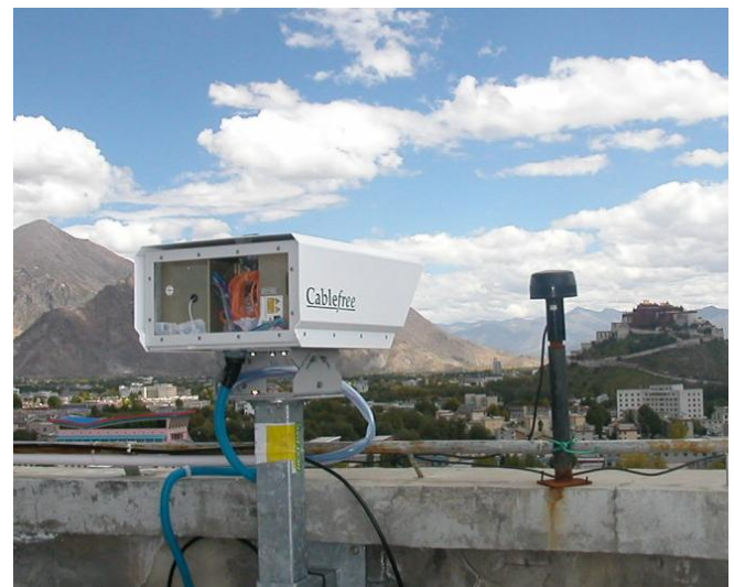
Parapet-wall installation of CableFree’s FSO takes a few hours, compared to days or weeks for cable/fibre digs.
